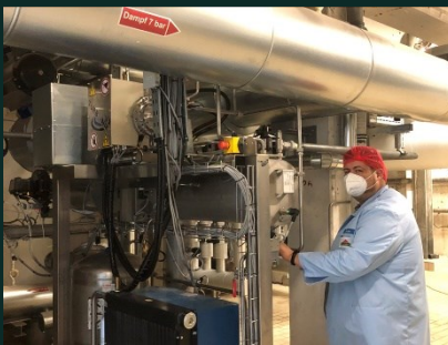
Schwarzwaldmilch Offenburg Pressure reduction instead of a control valve.
